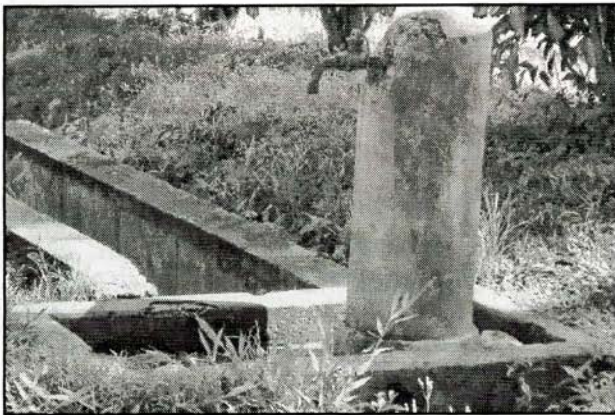
Figure 3: An example of a standpipe used by WASA for water distribution.
